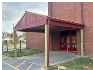
Walkway Covering - Large Gym
